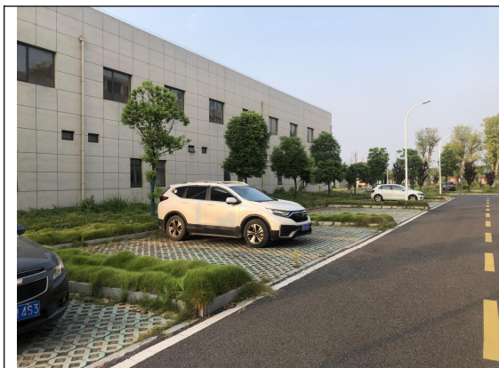
堆场区透水砖铺设
